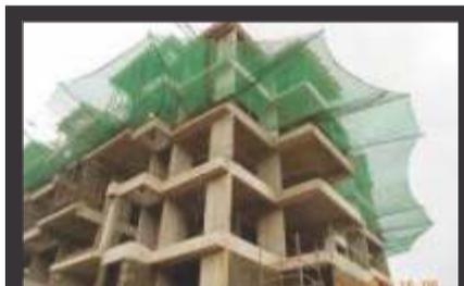
Safety nets and barricading so that edges from which people could fall are provided with double guard rails or other suitable edge protection.
